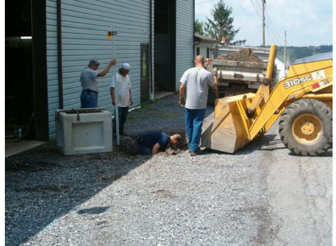
Washington Township crew prepares for paving.
